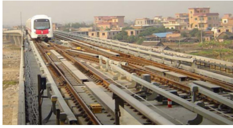
Fig. 2. The LIM elevated bridge of metro line 4.
