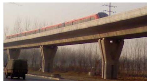
Fig. 1. The LIM elevated bridge of Beijing airport line.
